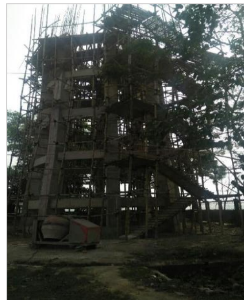
Figure 21 Construction of overhead tank in Bera
