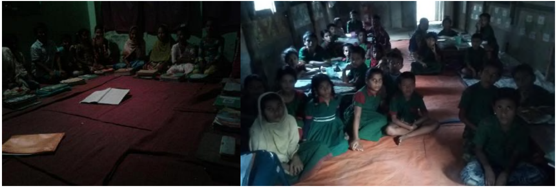
Figure S3: LCs with limited light and ventilation facility. Left: Halishahar (Chattogram), right: Tarail, Kishoreganj.
